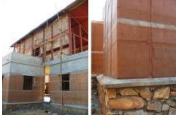
Image 22: Rammed earth walls raised on a stone plinth, wattle and daub panels on the upper floor (Hunnarshala, 2001)
