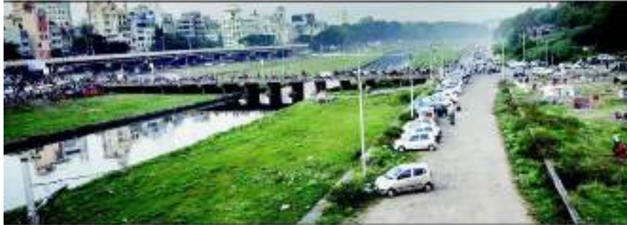
Fig 5: Channelization of Mutha River in Pune Source: Clicked for personal use
