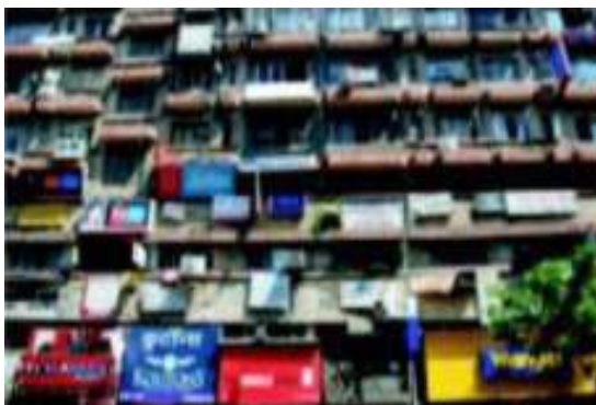
Figure 8: A forest of hoardings and signages with no visual relief - Karve Road Pune
