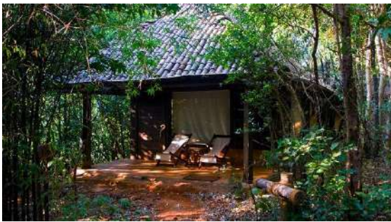
Figure 1: Cottage showing the use of Acacia wood and other sustainable materials in wildernest nature resort
