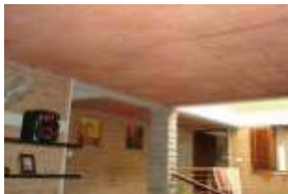
Fig. 12. Hourdi blocks as heat insulator
