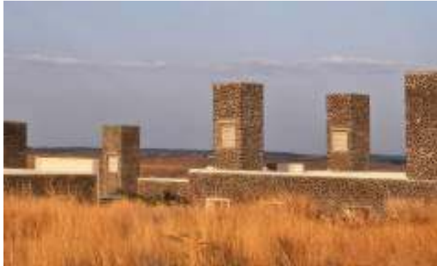
Image 24: Exterior view showing wind towers (Picture credits: RMA website)
