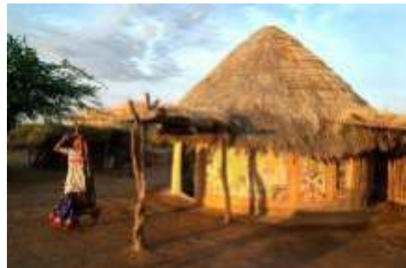
Image 16: Sloping timber roof of a bhunga covered with thatch and ornamented walls
