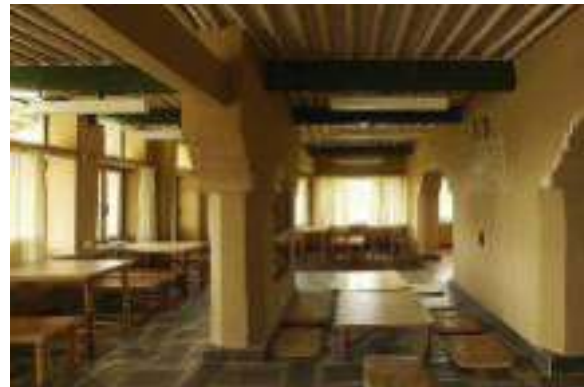
Image 8: Local slate, adobe and bamboo in Sambhaavnaa Institute, Himachal Pradesh, 2000 by Didi Contractor
