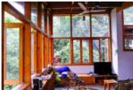
Fig. 7. Large reused windows
