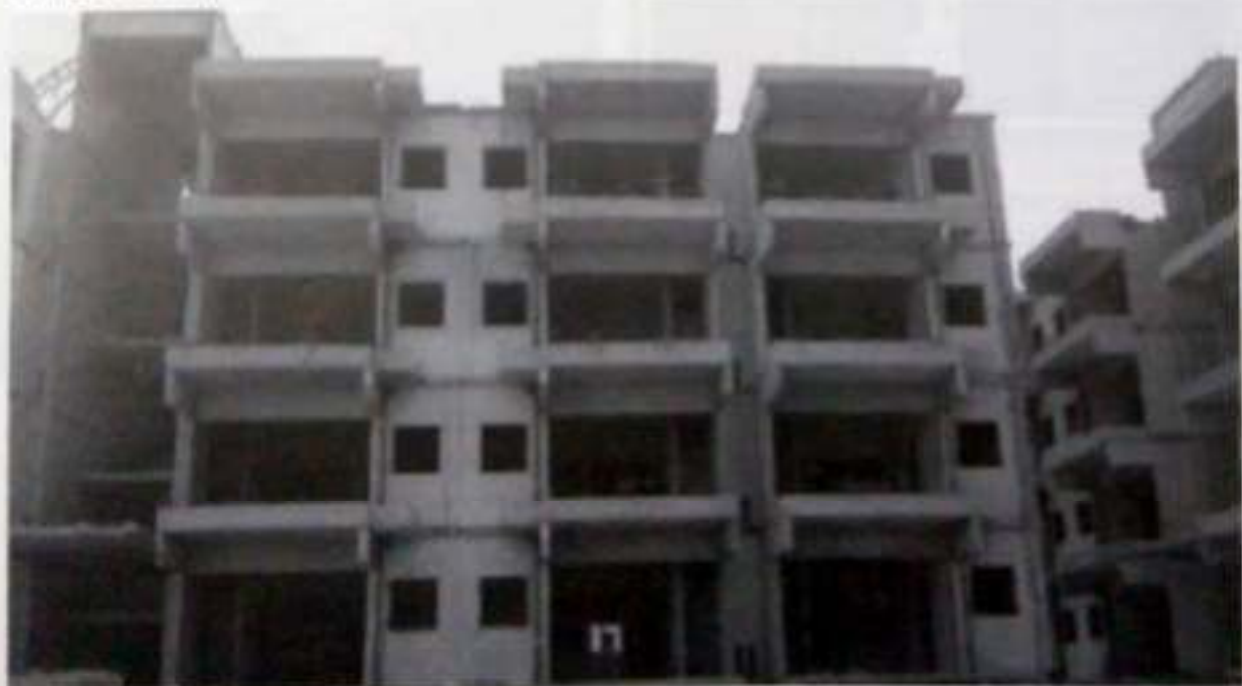
Fig 4: Mid rise precast panelled scheme of Bangalore (Source: NBM Media Publication, 2015)
