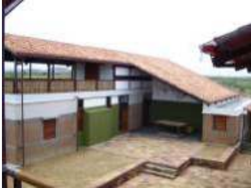
Image 21: Raised plinth connects the spaces; sloping roofs shade the top storey (Hunnarshala, 2001)
