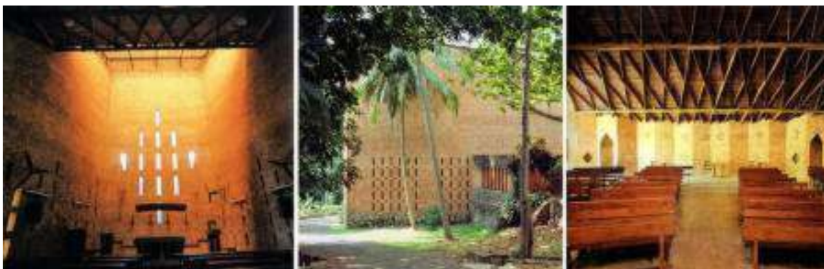
Image 23: Brick cavity walls with jaalis and wooden framed roof (Mehrotra , 2011)
