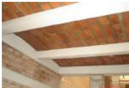
Fig. 11. In-situ Jack arch roofing panels
